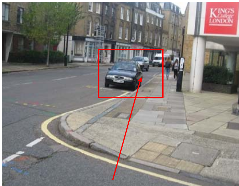
Figure 11: Obstruction of westbound visibility splay exiting Swan Street
