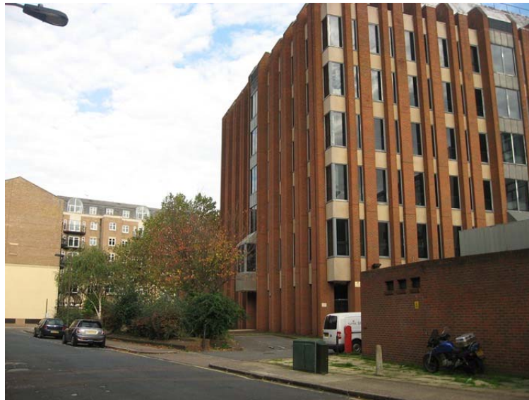
Figure 13: Large empty commercial property in Cole Street
